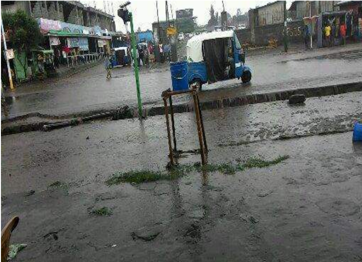
Figure 26. Photo taken during drainage ditch over flow (Left Side or besides of bus station Entrance)
